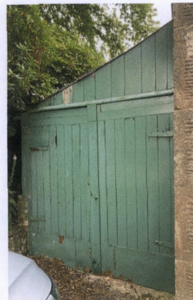
View of garage/ shed on gable.
