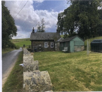
View of existing building from south east.
