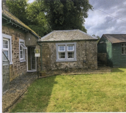
View of existing extension and shed.
