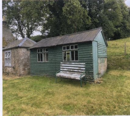
View of existing shed.
