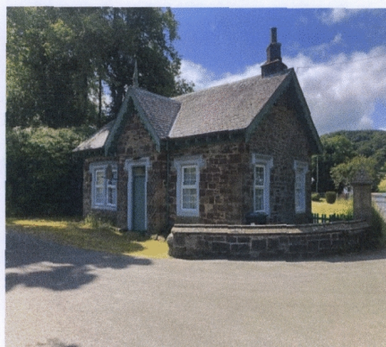
View of front elevation looking West.
