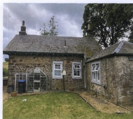
View of rear elevation and existing extension.
